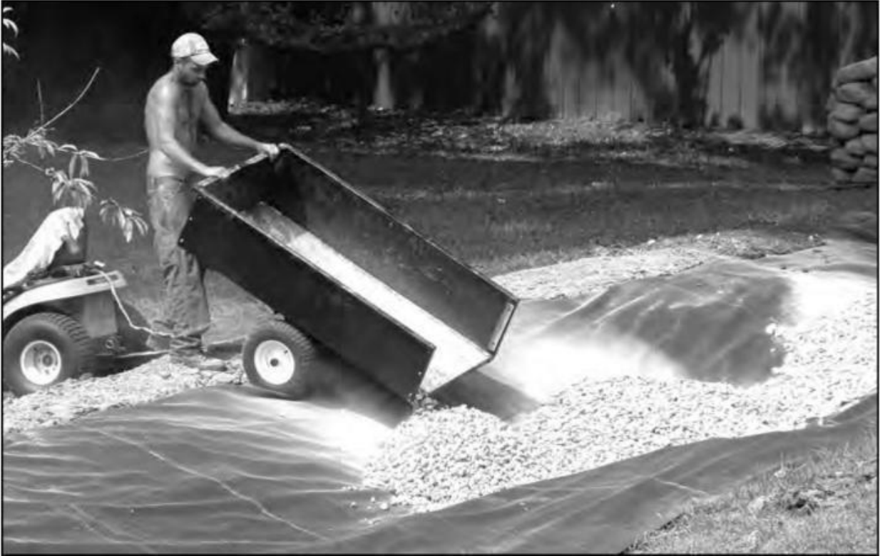
Rocks are being placed on top of the stream bed liner. Photo courtesy of Douglas R. Brown.
