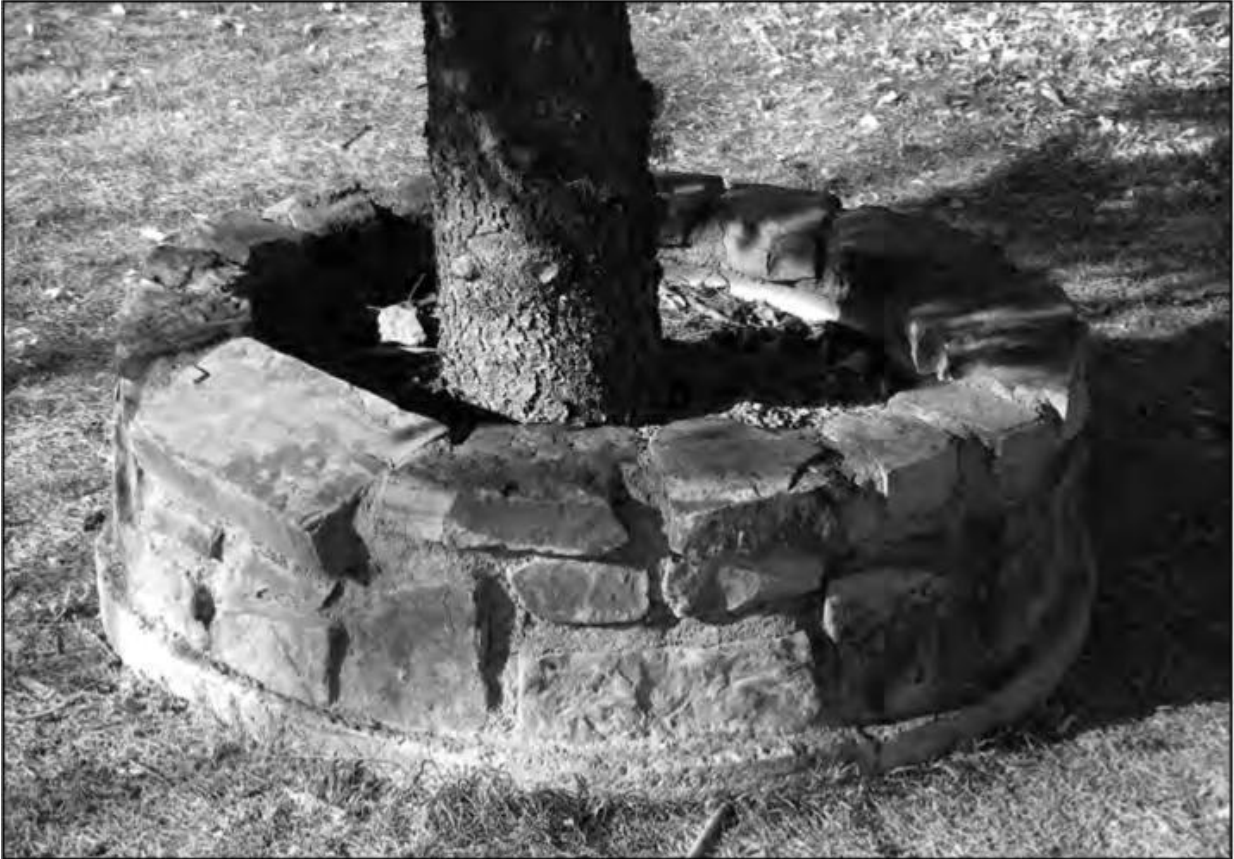
Field stones were used to create a small retaining wall around this pine tree.
