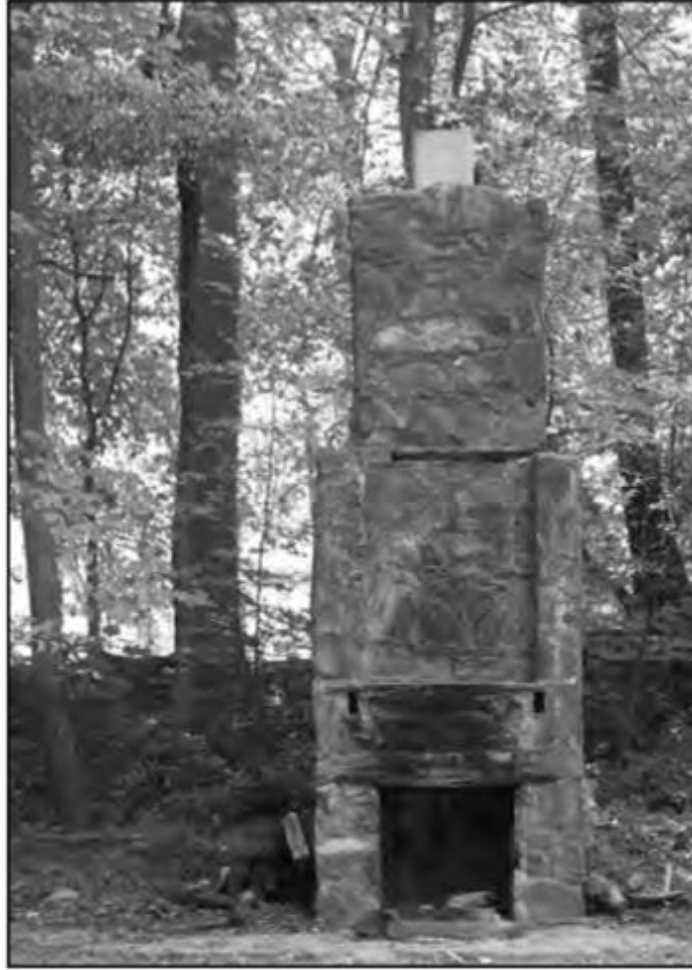
The stone fire pit and chimney above is constructed of slate.
