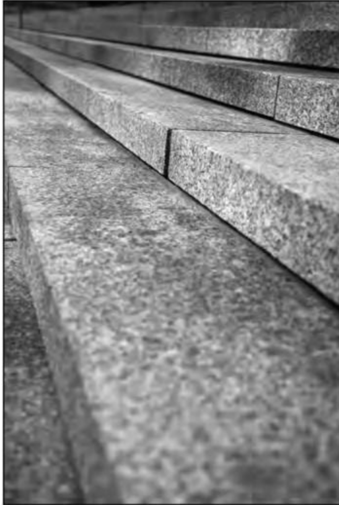
Close-up of granite steps.
