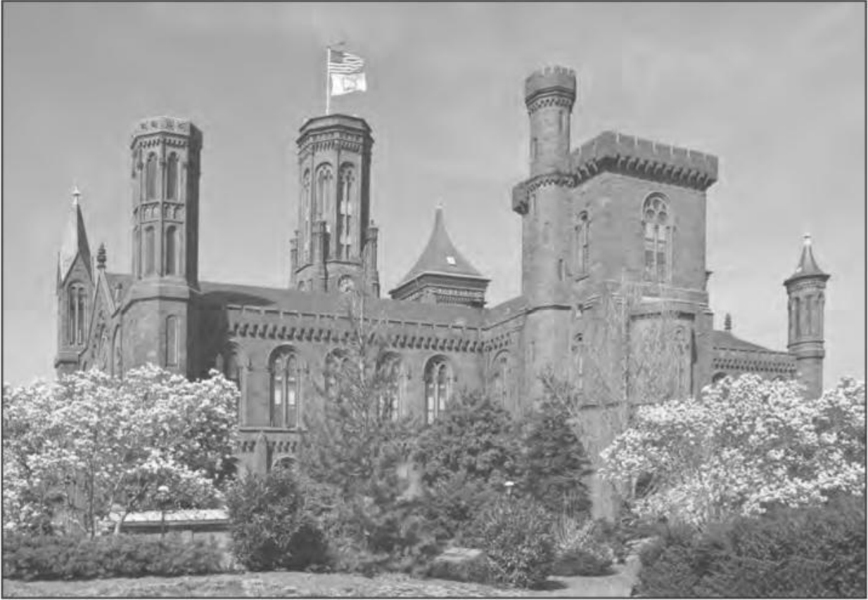
The Smithsonian Castle and Information Center was built out of red sandstone quarried from Seneca, Maryland.
