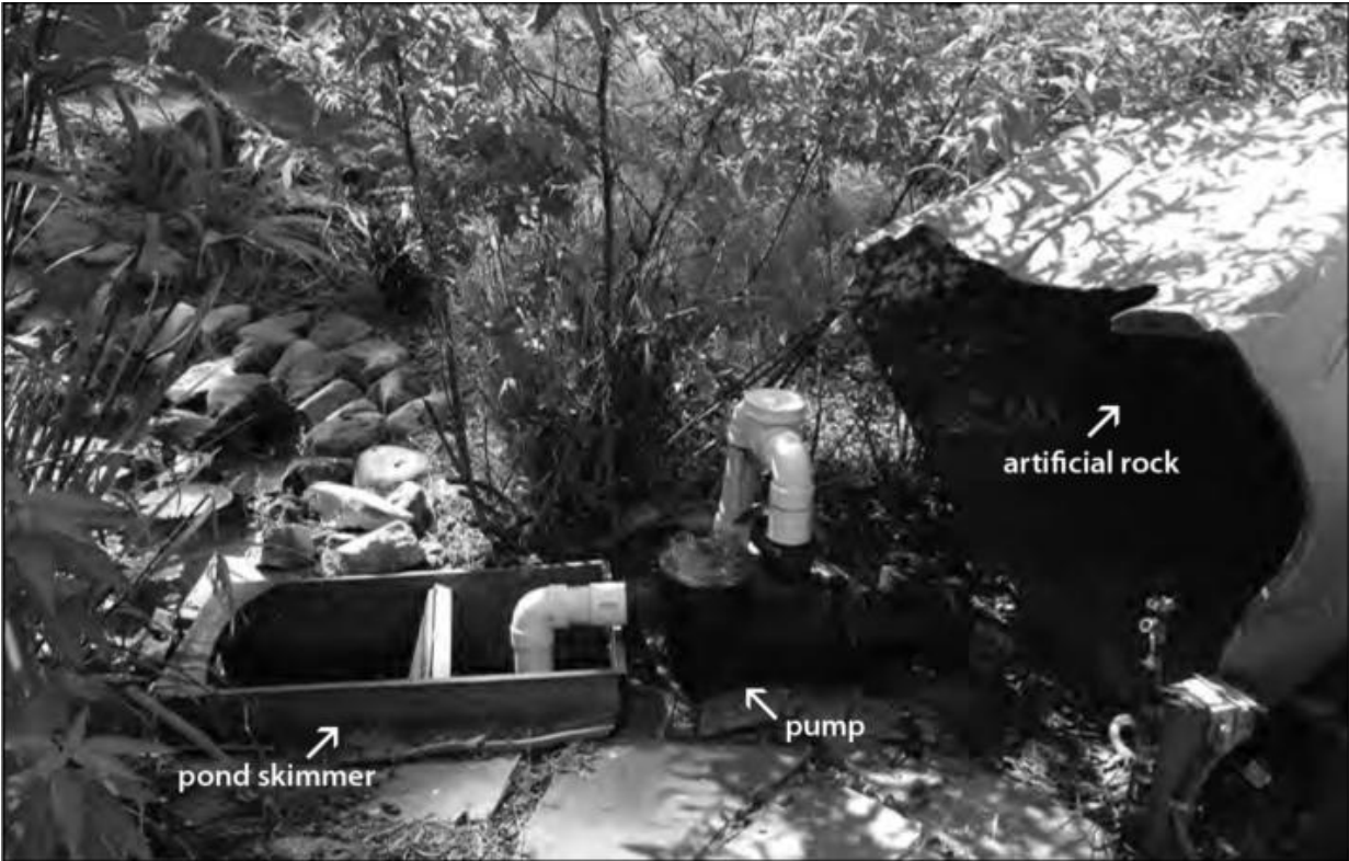
A pond skimmer and pump that is disguised by an artificial rock. Photo courtesy of Douglas R. Brown.
