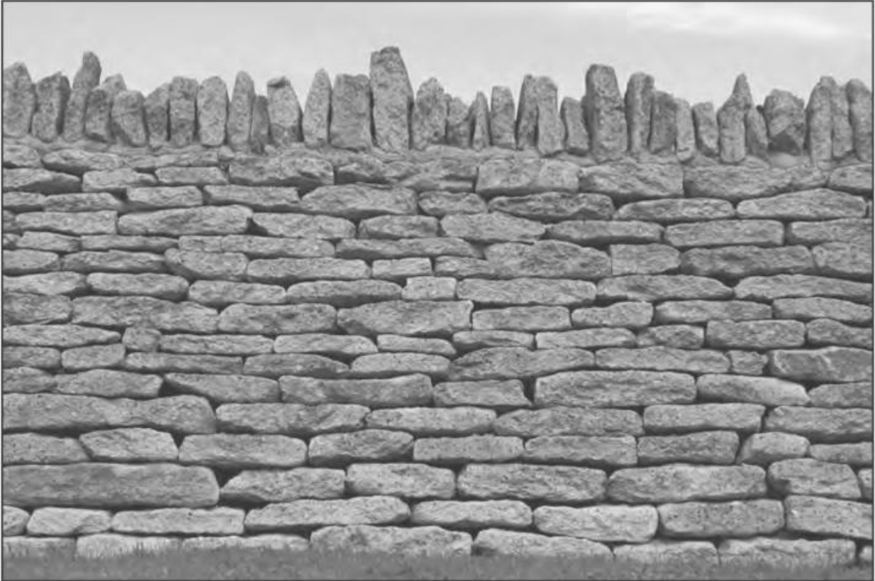
A dry stone wall at Batsford Church in Gloucestershire, England.
