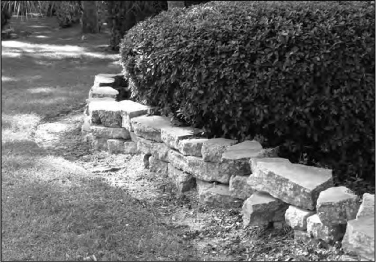
Here recycled concrete was dry stacked to create a small wall. Photo courtesy of Douglas R. Brown.
