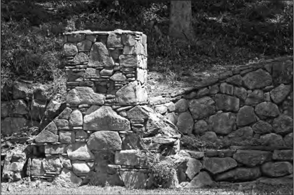
Barbecue pit that is made out of fieldstones and has a chimney.
